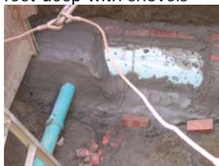
and buckets. Although we did not find the blockage on the inside, we were able to pinpoint the location in the street. We were also able to install a clean-out, which is required by code and will be very helpful in the future should this situation arise again.
